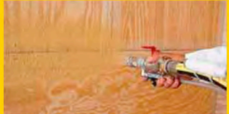
Spray Gold Fill® over the joints and spot fasteners
