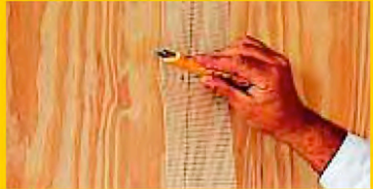
Mesh the joints
