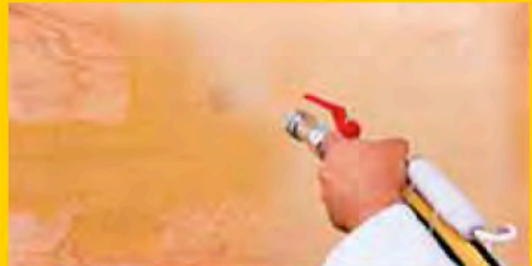
Spray Gold Coat® on the sheathing
